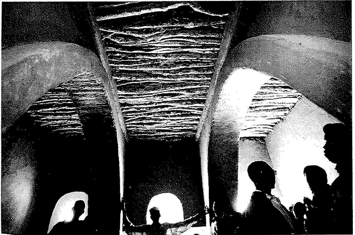
Long span arches
