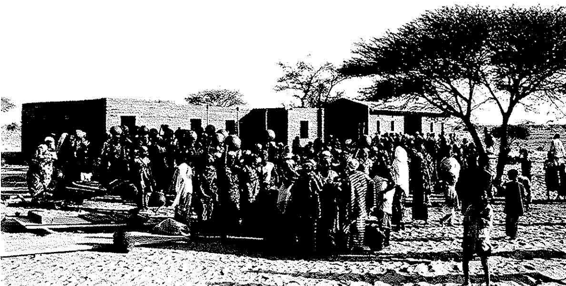
Health centre in Cake: every building is constructed with the active participation of the villagers
